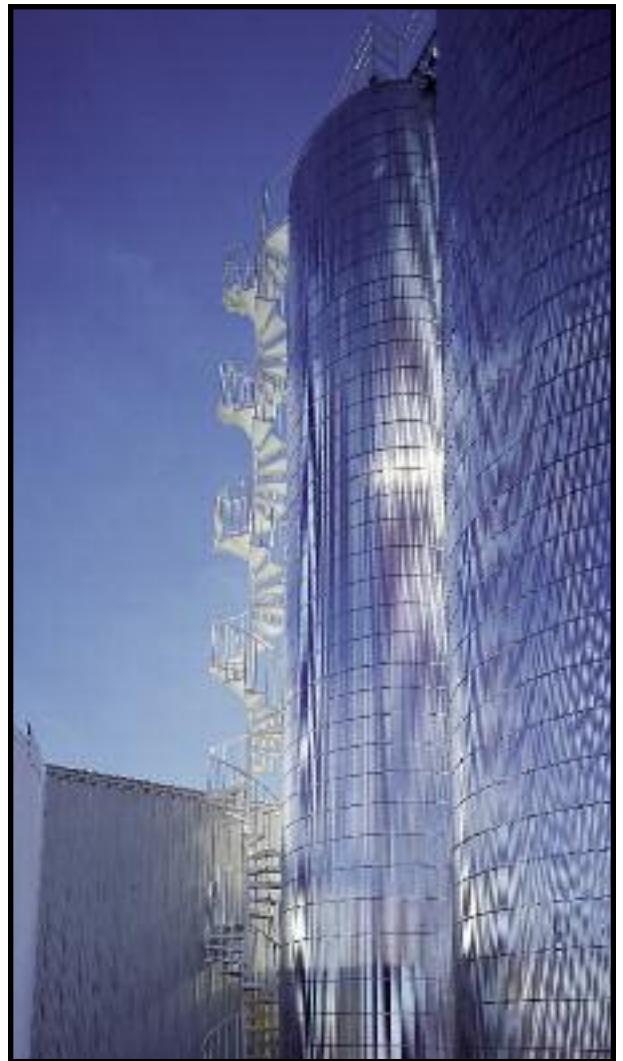
60S, 56' floor to floor, 1-1/2" Rd. handrail, 1" square baluster, checker plate treads, w rest landing
