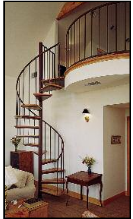
52S 1-1/2" Rd. handrail, 1" Rd. Balusters, #140 oak tread w/nose.
