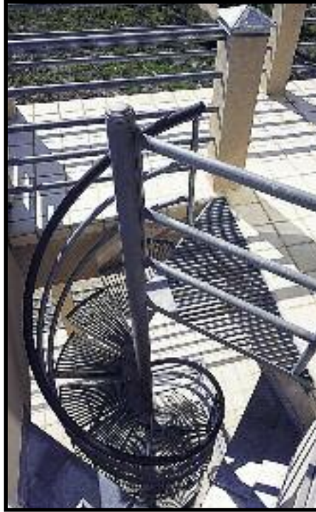
Radial grate tread and 90° triangular radial landing
