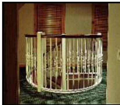
270° circular rail with #237 oak handrail, #326 balusters and 3" square posts
