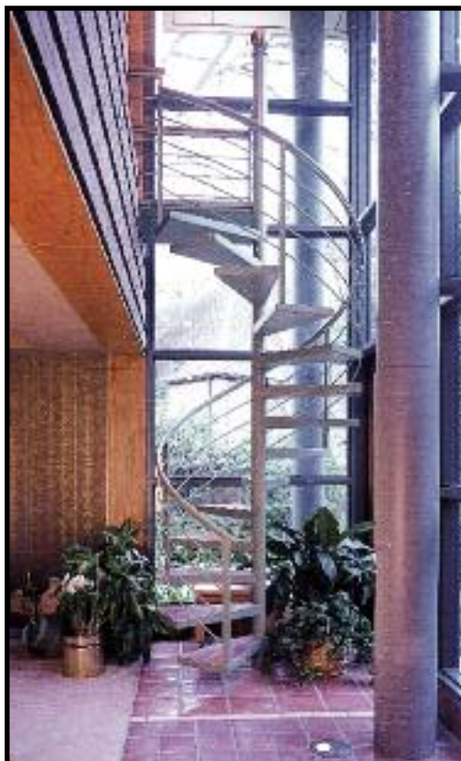
60S oval mahogany handrail, #326 baluster, #140 mahogany treads w/nose
