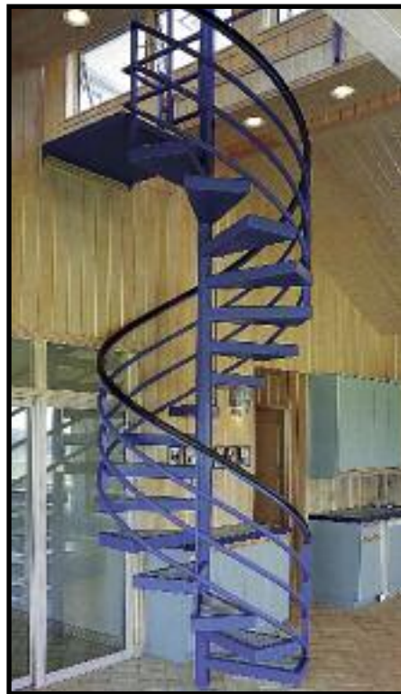
60AL aluminum 4 line rail, pan type tread, tile inlay by others
